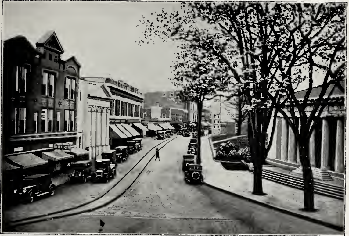
HIGH STREET, LOOKING WEST, WESTERLY
